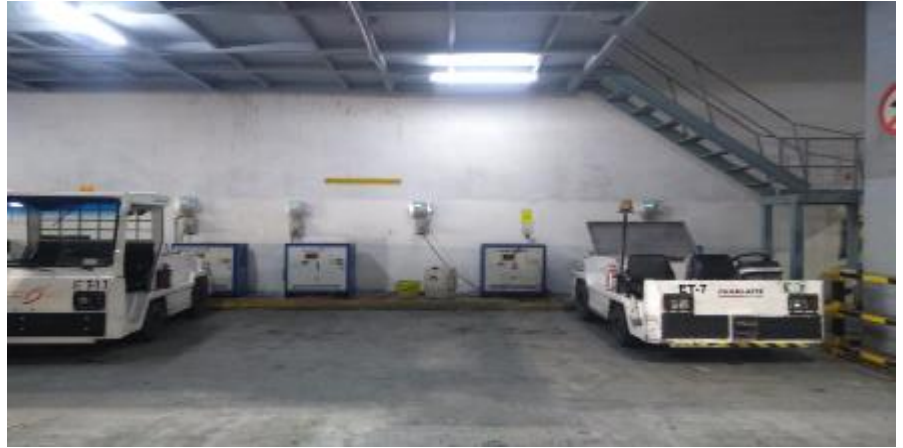
Installed 8 no's of 3-phase new Energy meters so that Energy Consumption can be recorded.
