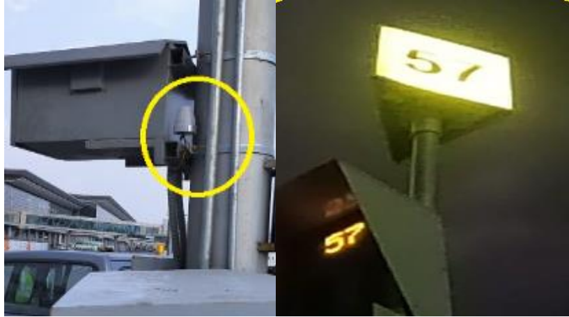
Installation of Photocell Sensor in Outdoor Signage Boards
