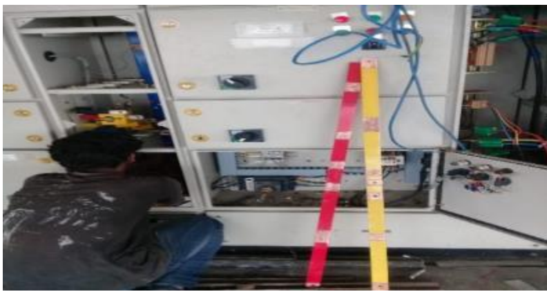
Redundancy Provision to ATC Panel
