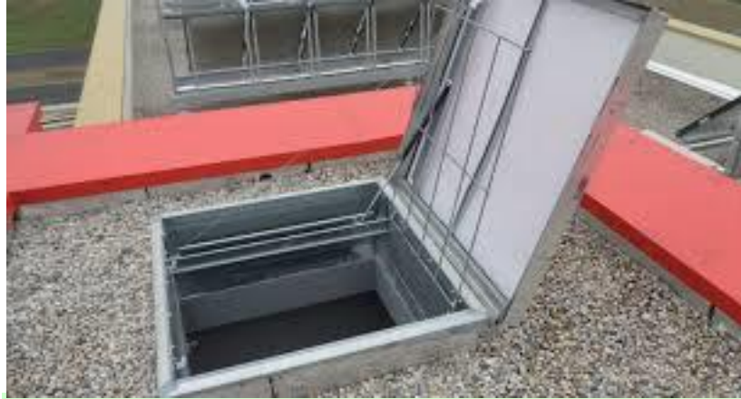
Smoke vent doors real time open & closed status integrated with IBMS.
